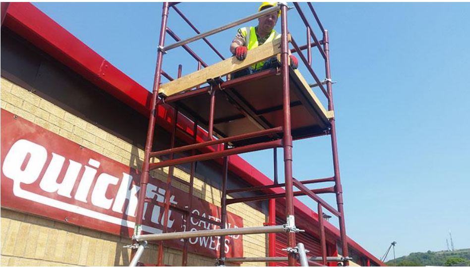
16. Fit the triple guard rails onto spigots as photo.
